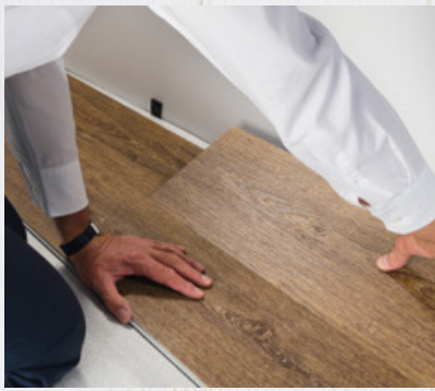
FIG. 4 Take another long plank (3). Repeating the previous step, insert the long side of plank (3) into the long side of plank (2). Then slide plank (3) to your left until the short side is in contact with the short side of plank (1).
