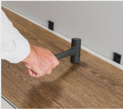
FIG. 6 Using a soft rubber mallet, slightly tap the joints on the short side to secure. This ensures 3x locking. Feel the seam with your fingers to make sure the seam is fully engaged.
