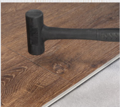
FIG. 8 As you go, don't forget to use a soft rubber mallet on the short sides to secure the locking. Be sure to check seams in the light to make sure you are not breaking the click from mis-alignment.
