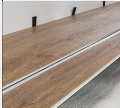
FIG. 10 Lift up the entire row in the same angle as you did during installation, then slide the rows apart.
