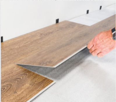
FIG. 7 Continue alternating planks on rows (1) and (2) to avoid misalignment. From row (3) onwards, installation does not require alternating rows. Install one row after the other by starting with angling on the long side, sliding until the short sides are in contact and then locking the short side.
