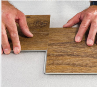
FIG. 11 Disassemble the row by sliding apart the planks on the short side. Do not pull straight up as the short side will be damaged.
