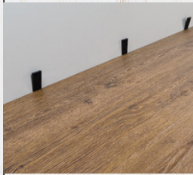
FIG. 9 When completed, pull all spacers and double check to ensure there is the required expansion gap..
